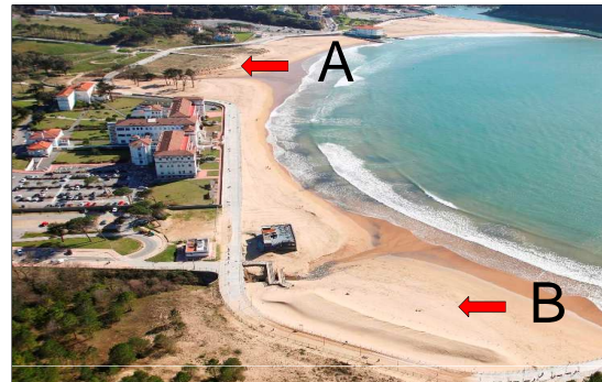
Figure 2. The sites after the restoration started
