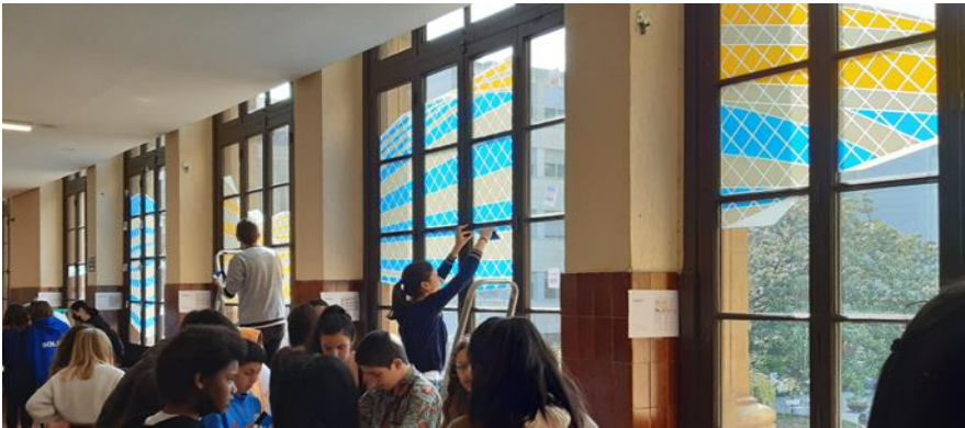
FIGURE 2. Installation of translucent vinyl on glass to investigate the science of light
