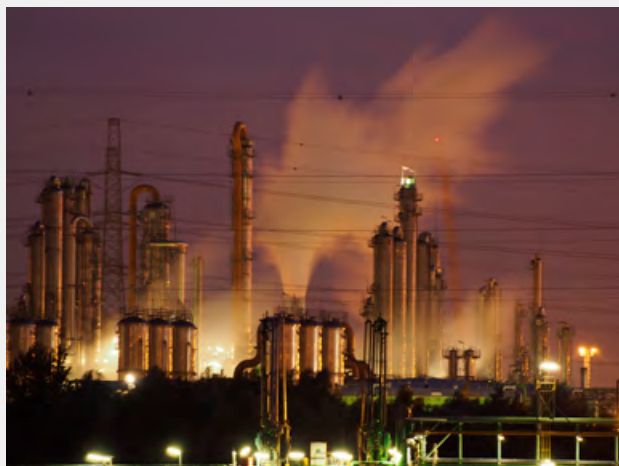
An INEOS plant in Belgium.
