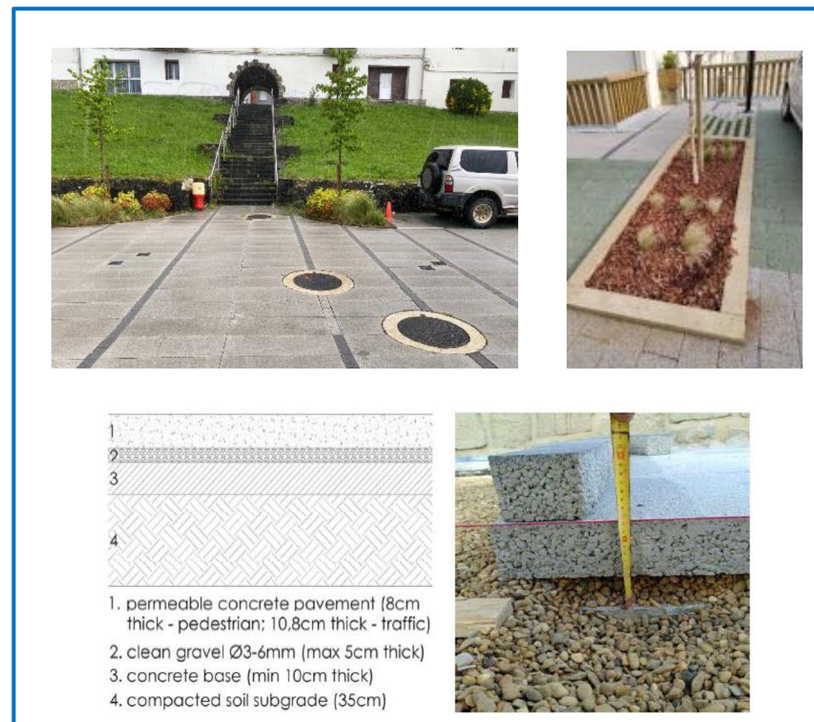
Parking permeable (1600 m 2 ); hormigón poroso (PC)
